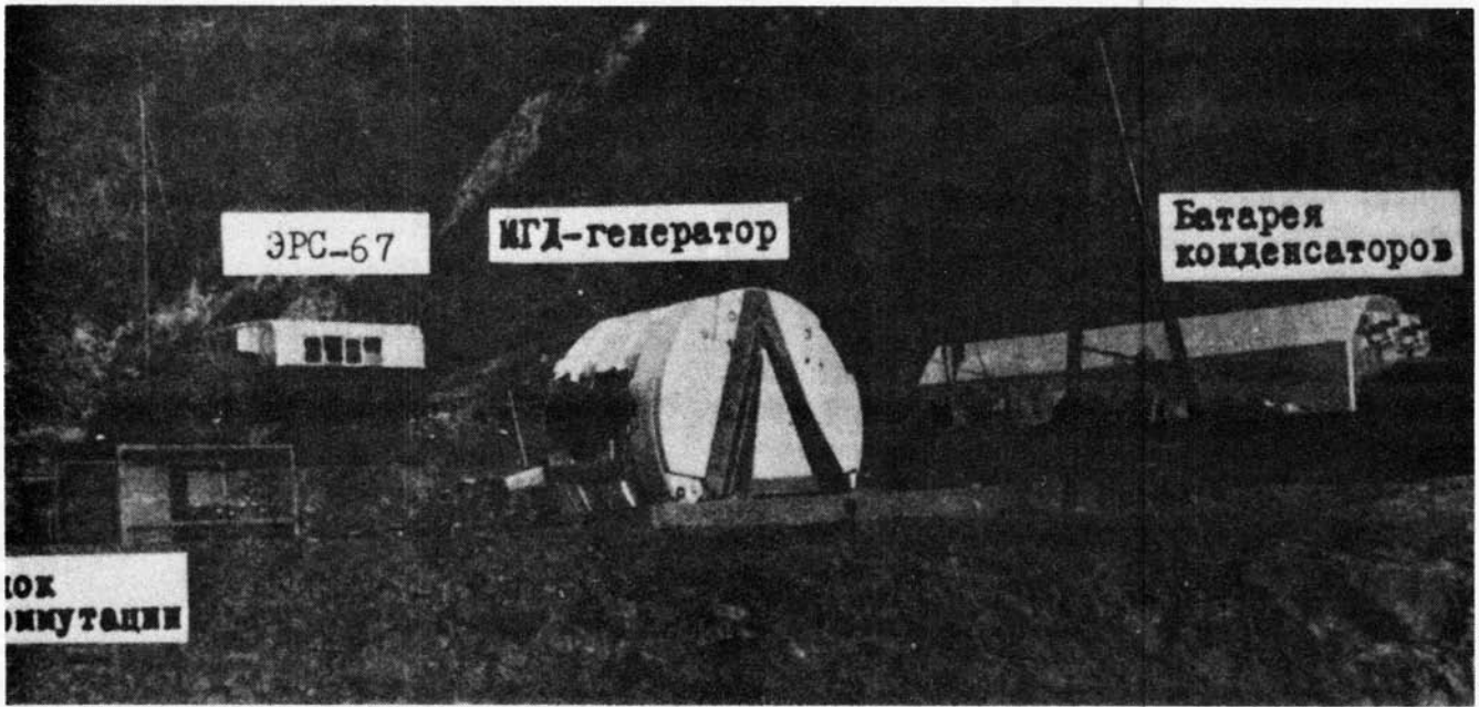
The Soviet Pamir MHD generator. Included in this photograph are the generator, the condensers, and other pieces of equipment on site in the Pamir Mountains. The MHD generator was moved by truck to various places in the mountains to do electromagnetic soundings for earthquake prediction.
