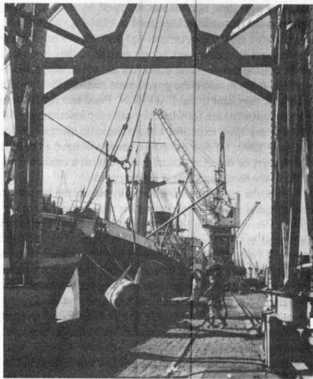
Cotton being loaded onto a Yugoslav freighter berthed at Port Sudan on the Red Sea. The cranes shown in the foreground were paid for by a World Bank loan. At the time this picture was taken—1962—the only technology Sudan had inherited from the British was related to cotton, the export crop promoted by colonial policy, while the World Bank refused to encourage any improvement in traditional rain-fed agriculture to grow food.
