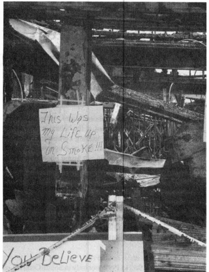
A building burned out in the Los Angeles riot—you can thank Warren Christopher, for one.
