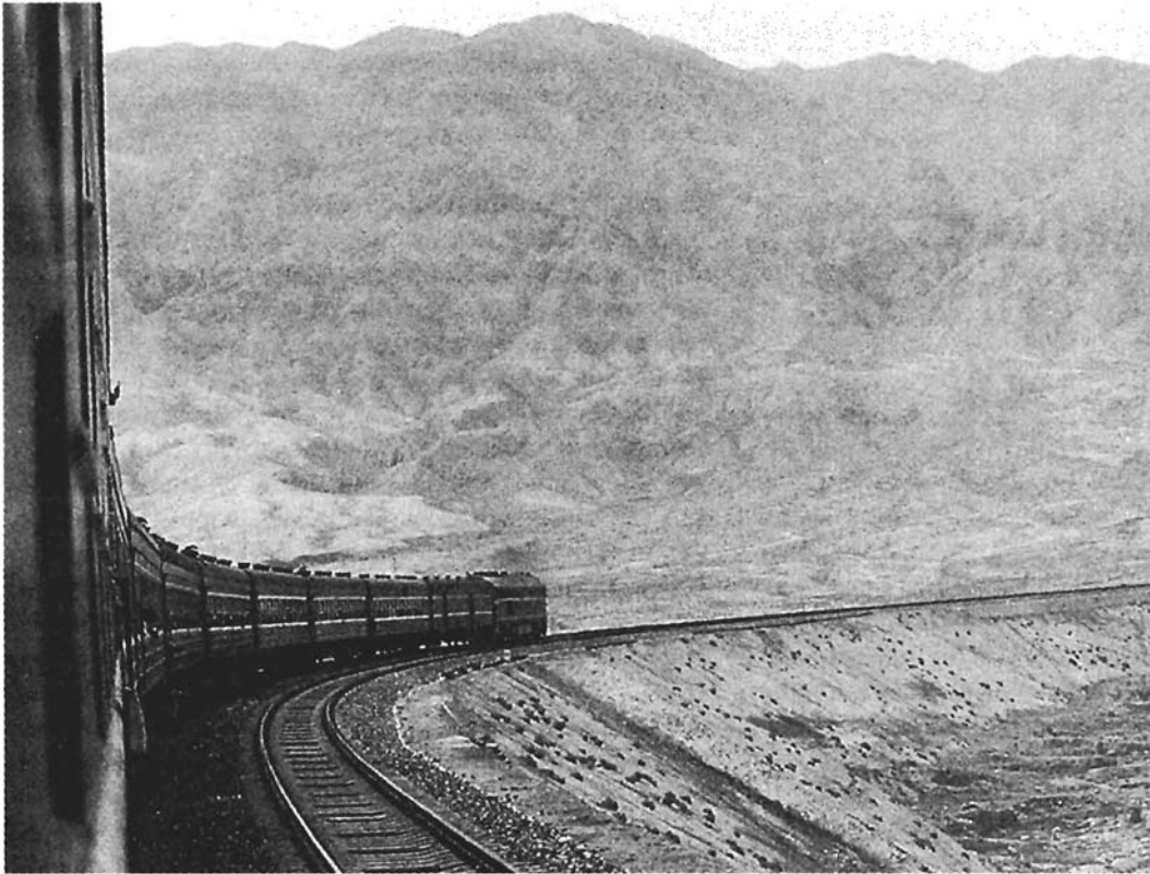
The main railway line in Lanxin in northwestern China.
