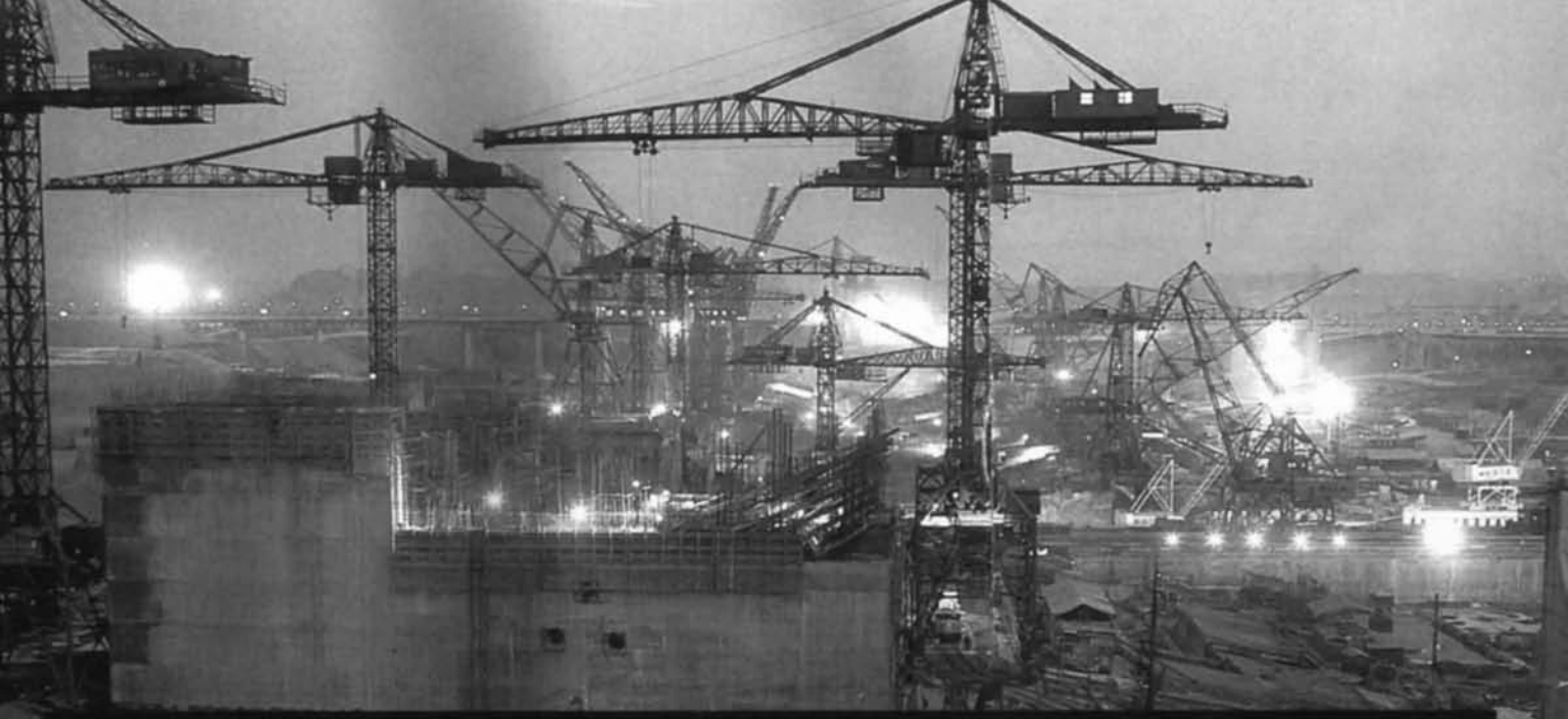
The construction of the Gezhou Dam in China.
