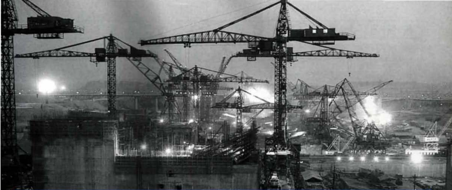
The construction of the Gezhou Dam in China.
