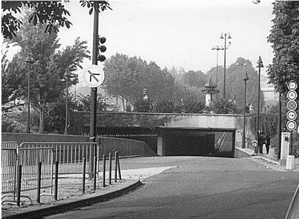
The entrance to the Place de L'Alma tunnel, as seen from the feeder road.
