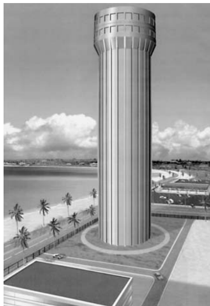
An artist's rendition of a modern seawater desalination tower. The structure houses a multi-effect distillation process (vertically stacked evaporators), for large-scale output (284,000 cubic meters daily).
