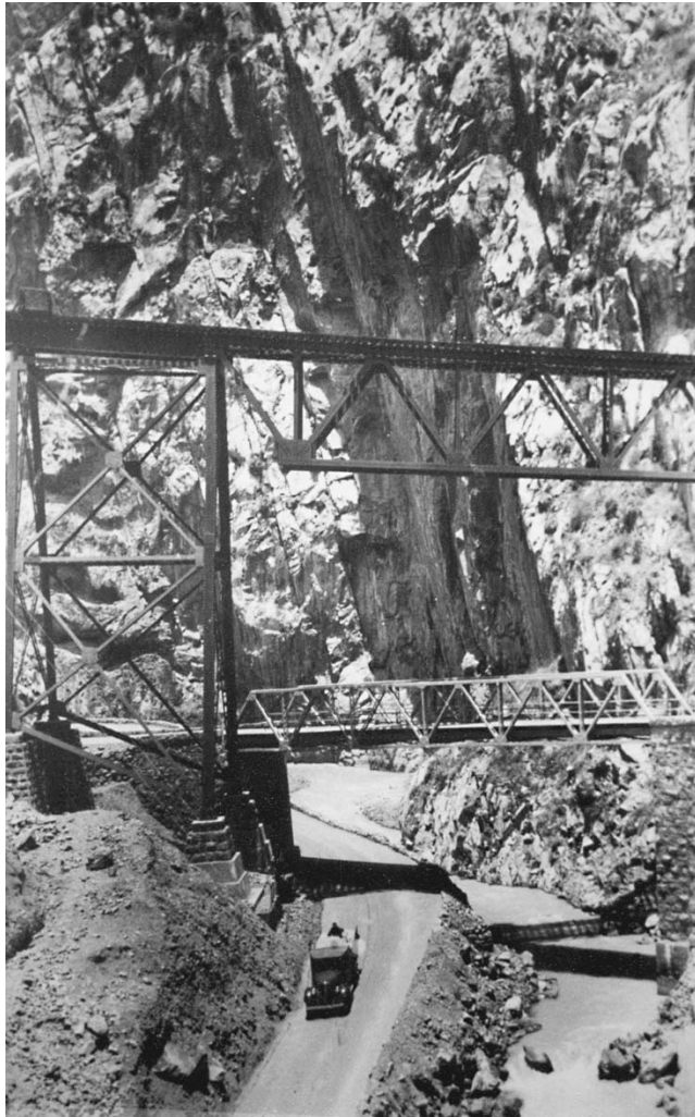
El Infeirnillo Bridge in the Andes Mountains, built by American engineer Henry Meiggs in the 19th century.
