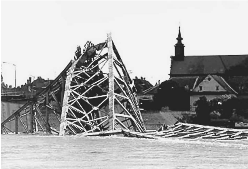
The Petrvaradin Bridge in Novi Sad, Yugoslavia, destroyed by NATO bombing in 1999. The Danube, the most important European waterway, must be cleared of the rubble of destroyed bridges and made navigable again.
