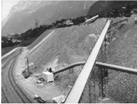
The approach to the Gotthard tunnel in the Swiss Alps.
