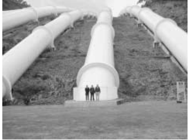
The six pipes of power station Tumut 3 are each 487 meters long, 5.6 meters in diameter, and collectively contain 10,260 tons of steel.
