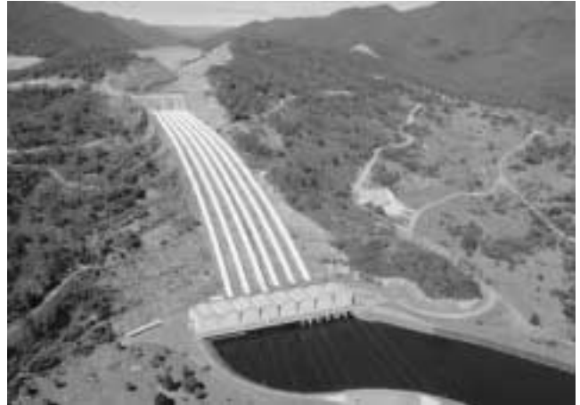
Two of the six generators at Tumut 3 power station can provide enough electricity to power a city the size of Australia's capital, Canberra.
