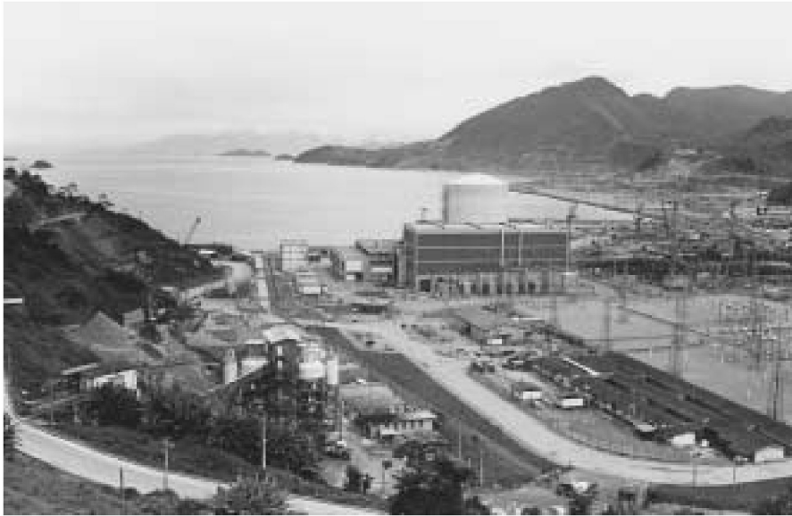
Brazil's Angra II nuclear plant. Development of Brazil's high-technology capability including nuclear power, was sabotaged by the international Malthusian oligarchy.
