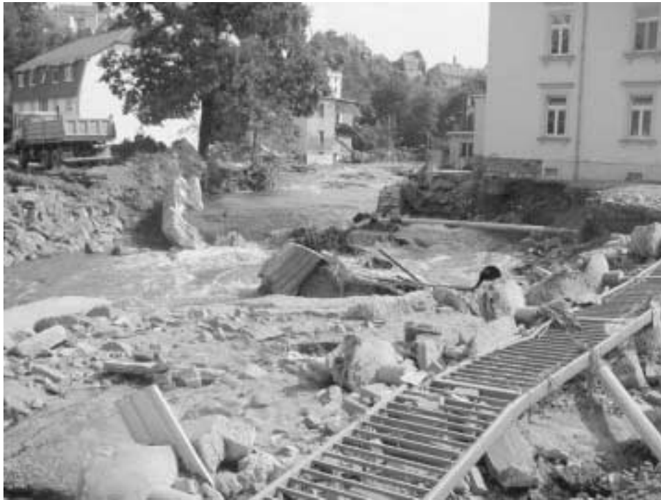
Flood damage in the German town of Dohna, in Saxony. The floods of 2002 were the worst in at least 160 years, and pose the necessity not only for rebuilding what has been destroyed, but also for launching the LaRouche Program for the Eurasian Land-Bridge: high-technology corridors of industry and agriculture built around high-speed rail and maglev networks.
