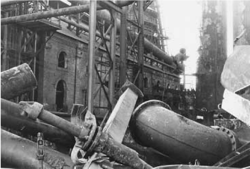
Demolition of a steel mill in McKeesport, Pennsylvania, in 1985. American populists cut their own throats by supporting free trade and deregulation, in the interest of getting a “cheaper deal.” The result: no U.S. economy!
