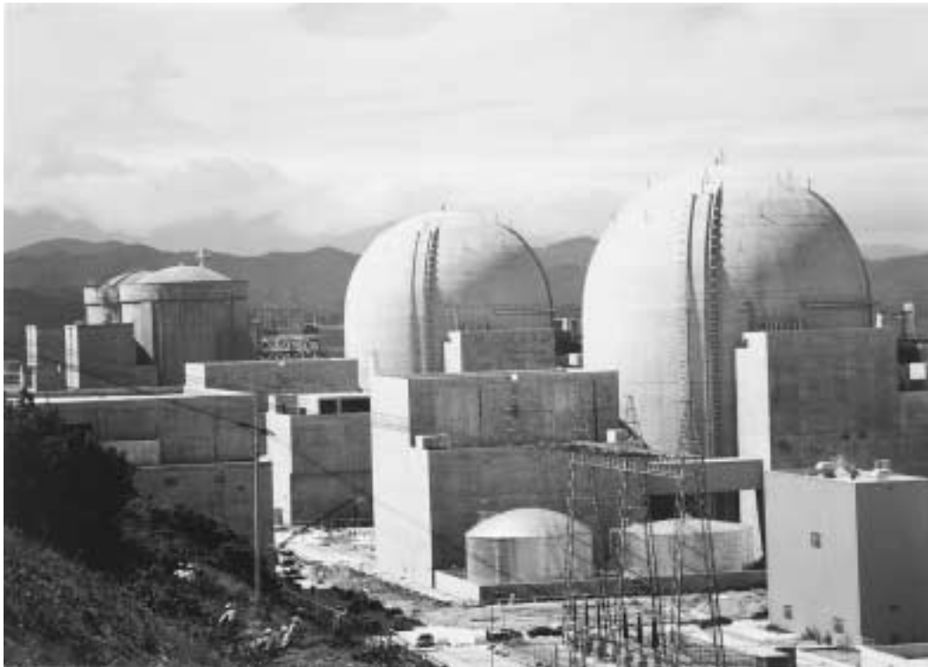
The Ulchin site, which has the first two Korean standard nuclear plants in operation, and two units under construction.
