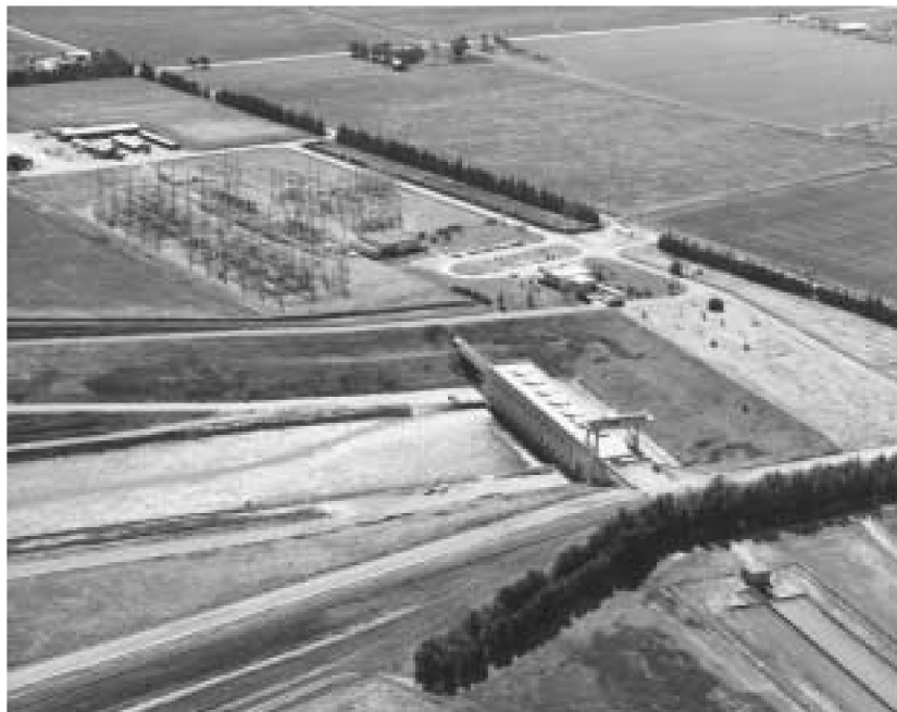
The Tracy Pumping Plant near Tracy, California, lifts water to the dry San Joaquin Valley. Water infrastructure development programs, a “NAWAPA-Plus,” can make the Great American Desert bloom as well, in the interests of both the United States and Mexico.
