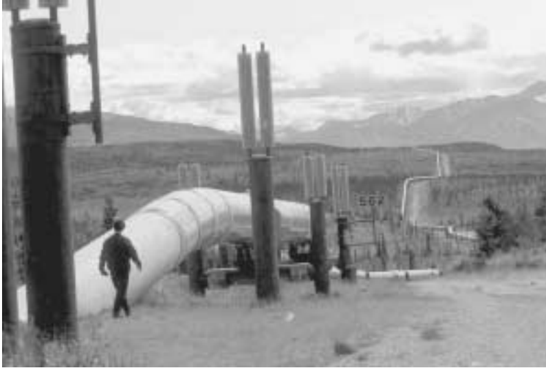
Pipeline to Alaska.
