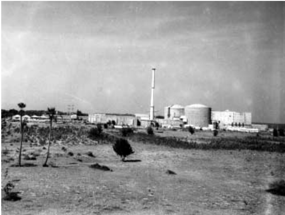
The Madras Atomic Power Station at Kalpakkam, India, includes a Nuclear Desalination Demonstration Project. Contrary to the narrow perspective of most conference participants, desalination is a vital technology to supply water for agriculture, especially in populous nations of Eurasia.
