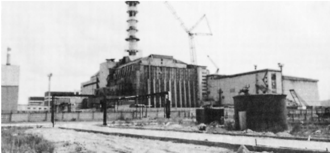
The damaged Chernobyl plant in 1992. The accident led to the first in-depth study of the long-term effects of low-level nuclear radiation, carried out by UNSCEAR.
