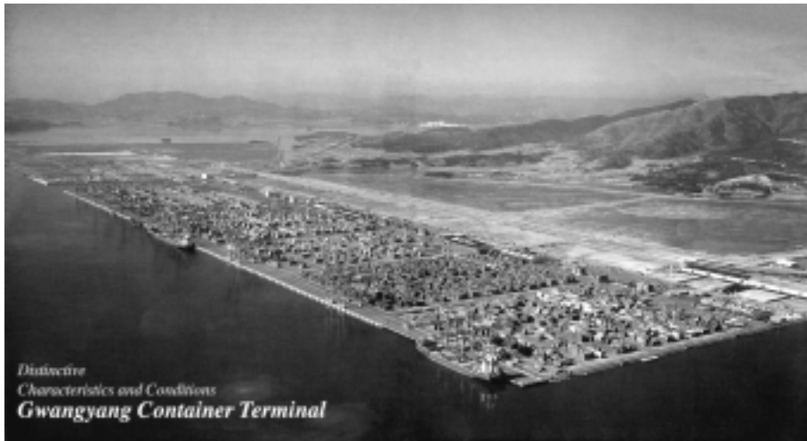
Korea's newest port will triple the nation's South Coast freight capacity, and serve as a "Gateway of the Iron Silk Road" which will connect through Trans-Korea rails to the continental railways of Russia, China, and Europe.
