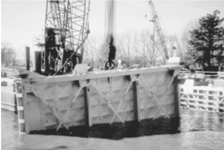
The crane “Quad Cities” here lowers into position a temporary gate, in the lower gates of the main chamber at Lock and Dam 15, on the Mississippi River, in Rock Island, Illinois, to replace a cracked structure removed for repairs off-site. This is the last temporary gate the Army Corps of Engineers has available for emergency use on the Mississippi.
