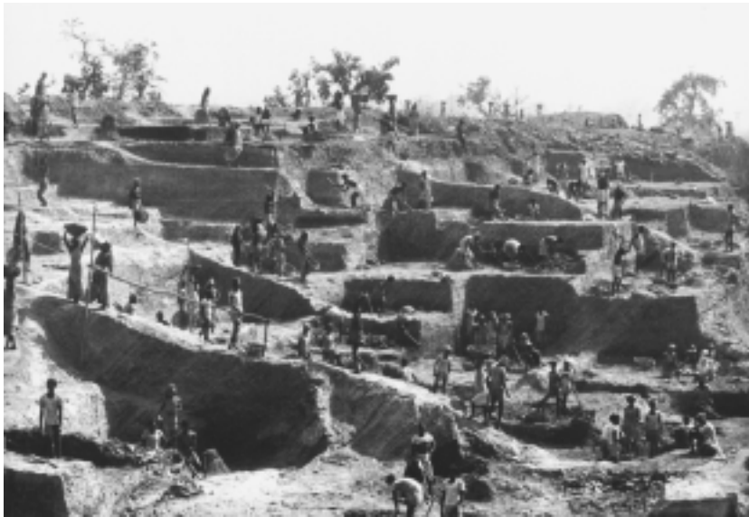
A World Bank labor-intensive coal-mining project in Digwadih, India. "The great mass of poverty in those leading nations of Asia, for which no clear remedy is yet in view, must touch the conscience of the world."
