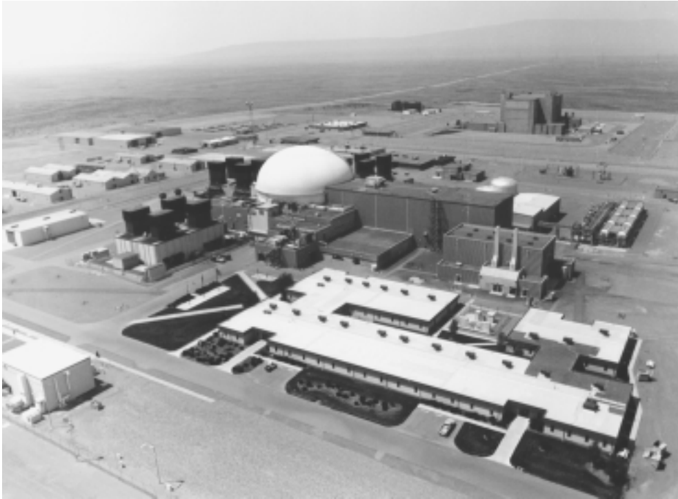
The Fast Flux Test Facility at Hanford, near Richland, Washington. The white dome is the containment building for the 400-megawatt multipurpose test reactor.
