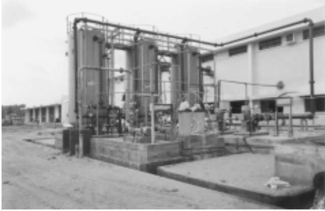
The sabotage efforts delayed, but did not stop, nuclear desalination. This 1,800 cubic meter/day nuclear-powered desalting plant is in Kalpakkam, India, a project of the Bhabha Atomic Research Center, and there are several projects on the drawing boards in other countries.
