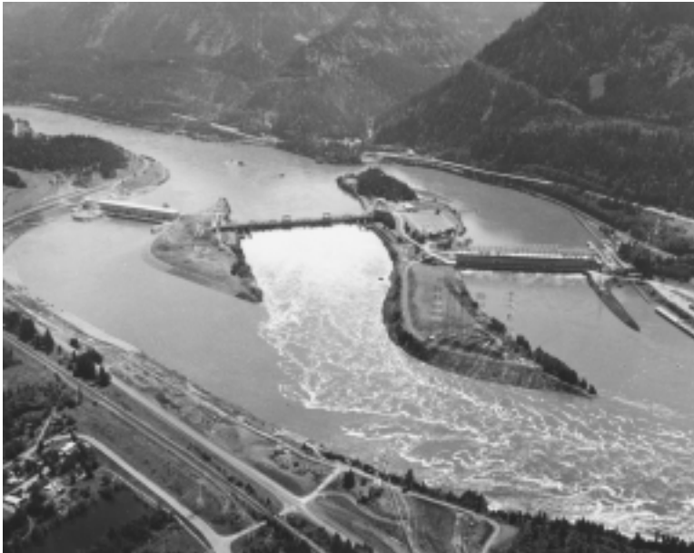
We urgently need to rebuild our water system, and we could immediately begin with the small water projects. “We can do those right away,” said LaRouche. Here, the Bonneville Lock and Dam project on the Columbia River, between Washington and Oregon.
