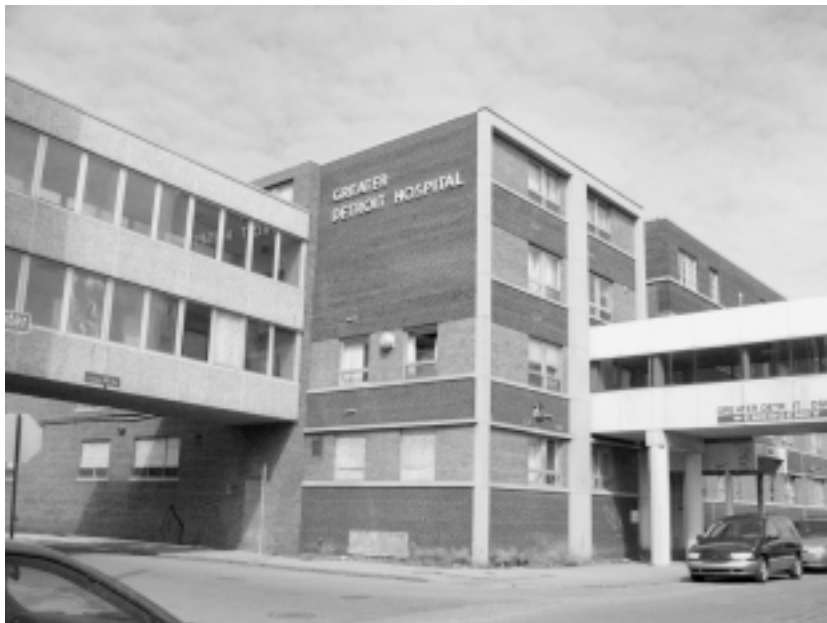
"As long as you maintain the HMO system, your idea of promising health care is a fraud," said LaRouche. "We are destroying the source of health care! How many hospitals have been shut down in the United States since 1973?" The Greater Detroit Hospital, shown here, is one of those which has been shut down.
