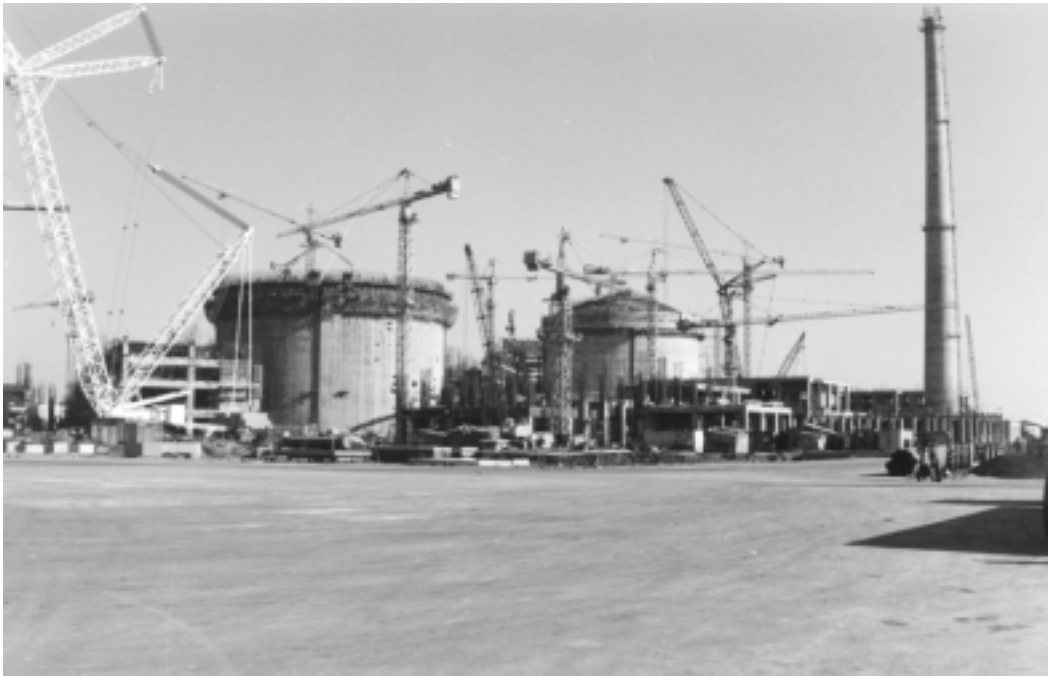
The first of India's pressurized heavy water reactors, a 540-MW unit, located at Tarapur. A second unit will be commissioned there this year.
