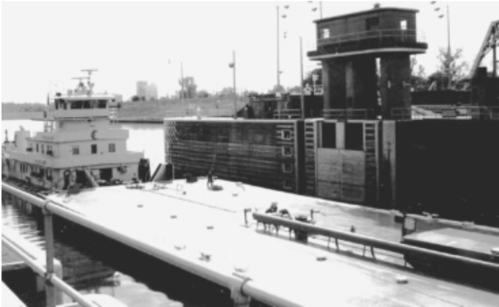
A fuel oil tow passes through McAlpine Lock and Dam on the Ohio River at Louisville, Kentucky. The lock was closed for emergency repairs last Summer.
