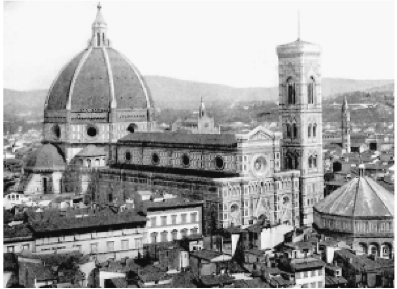
The Fifteenth-Century Renaissance built on the Classical method of science and statecraft of Nicholas of Cusa. Here, Brunelleschi's dome on the Cathedral of Florence, for which construction Brunelleschi made use of the physical principle of the catenary.
