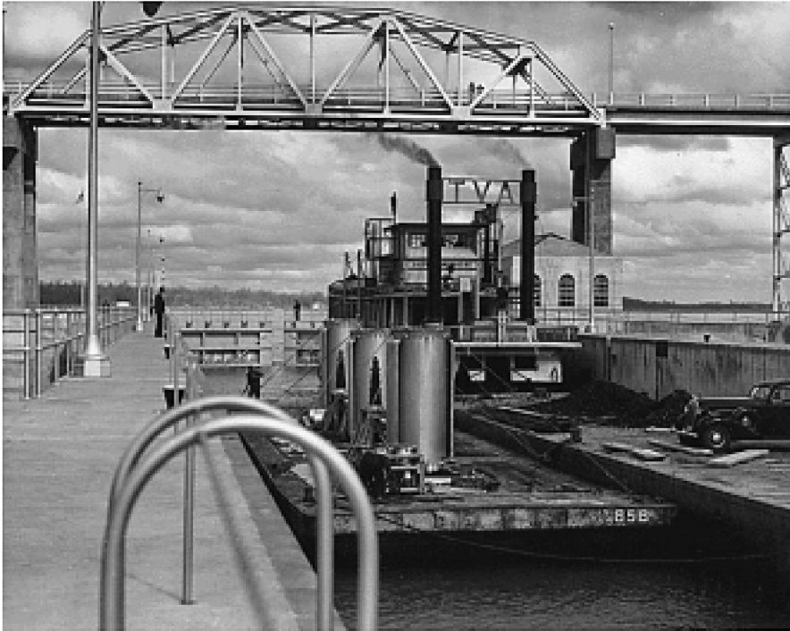
The Wheeler Dam navigation lock in Tennessee in 1942, constructed by Roosevelt's Tennessee Valley Authority. This was the first of eight dams that the TVA constructed on the Tennessee River. The Federal government provided the credit for these massive infrastructure projects, to get the economy moving again.
