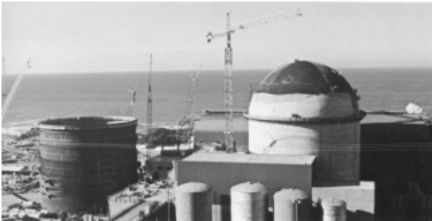
In the 1970s, the Pittsburgh-Des Moines Steel Company was a major manufacturer of aerospace and aeronautics test facilities, buildings, and bridges, and pressure vessels and structural components for nuclear power plants. Their nuclear manufacturing facilities, which no longer exist, built the containment vessel for the TVA's Browns Ferry nuclear plant in Alabama (shown at the top under construction), and both containment vessels for California's Diablo Canyon plants (bottom). In 1973, it was involved in 27 nuclear power plant projects.
