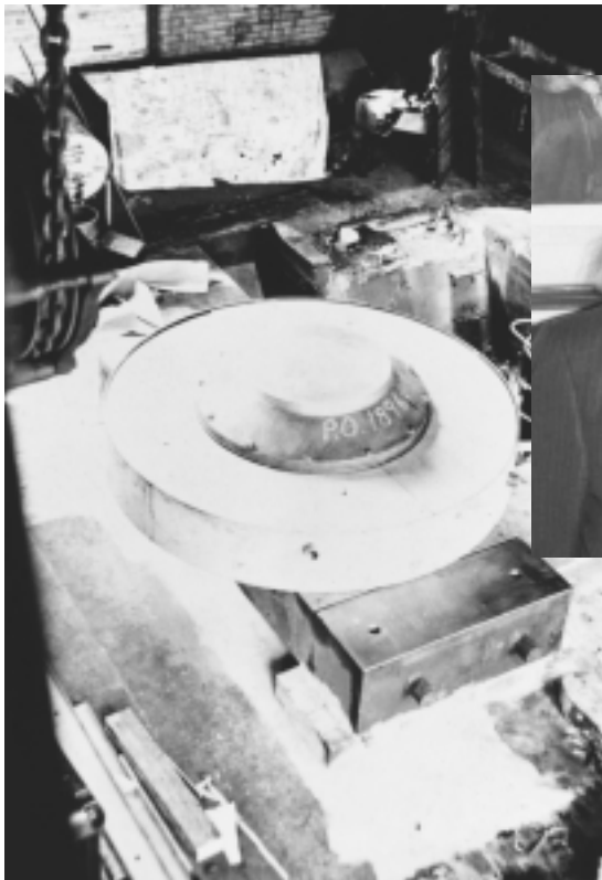
The half-assembled Chicago cyclotron magnet. This cyclotron, the second in the world, was designed and built by the late Dr. Robert Moon and a team of students of Dr. William Harkins at the University of Chicago in 1936. Inset: Dr. Moon in 1986.
