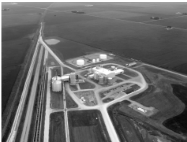
The Voyager Ethanol Llc plant, in Emmitsburg, Iowa. Note the rail cars, as well as roadways. Ethanol cannot be conveyed by pipeline. This is one of 50 plants in Iowa, either operating or under construction.
