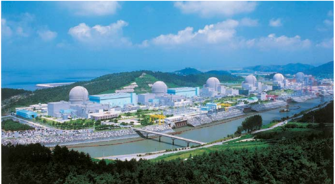
Korea Hydro & Nuclear Power Co., Ltd.
