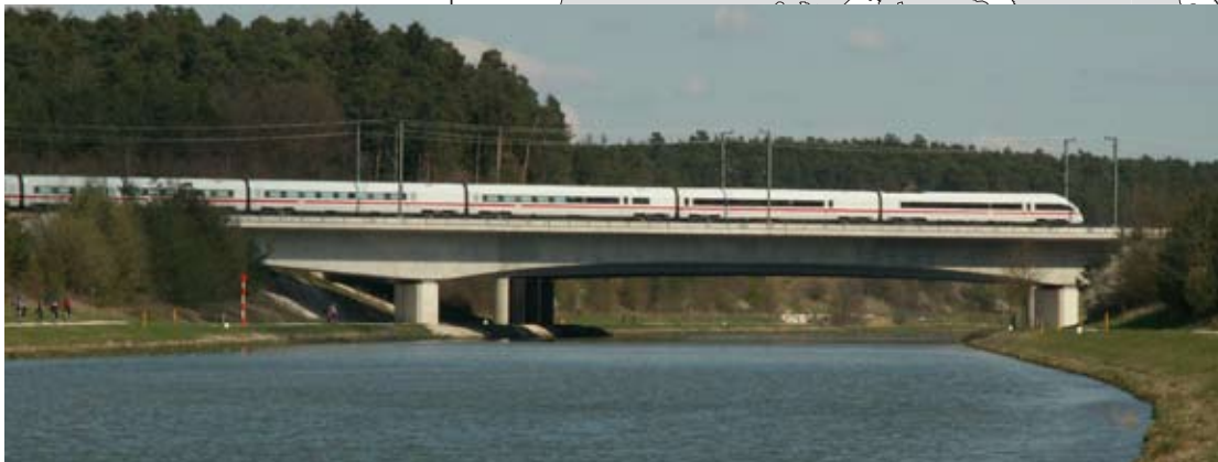
The Rhine-Main-Danube canal bridge of the Nuremberg-Ingolstadt high-speed rail line.
