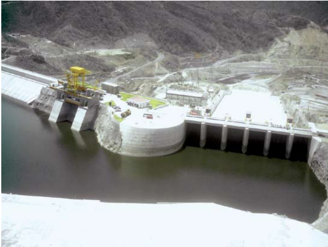
Each dam in the PLHINO project will require concrete, steel, gravel, sand, water, and a lot of both skilled and unskilled labor. Shown: a panoramic, photo of the El Cajón dam, in the state of Nayarit, Mexico.
