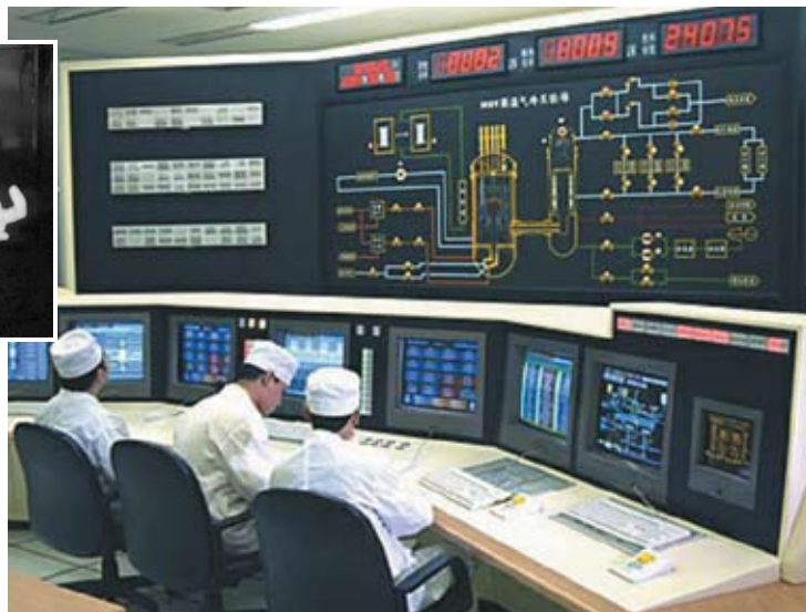
Chinese technicians in the control room of the experimental HTR-10, which has a pebble-bed design. China plans to construct a commercial-size 200-megawatt HTR starting in 2009.
