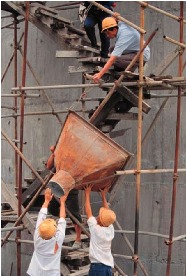
Workers constructing China's Three Gorges Dam, now the largest source of hydroelectric power in the world. The dam is a useful project, but it's not enough for a country the size of China.
