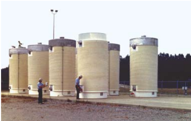
Dry casks of spent reactor fuel, stored on a concrete pad at a nuclear power plant. Why not reprocess it and burn it up?
