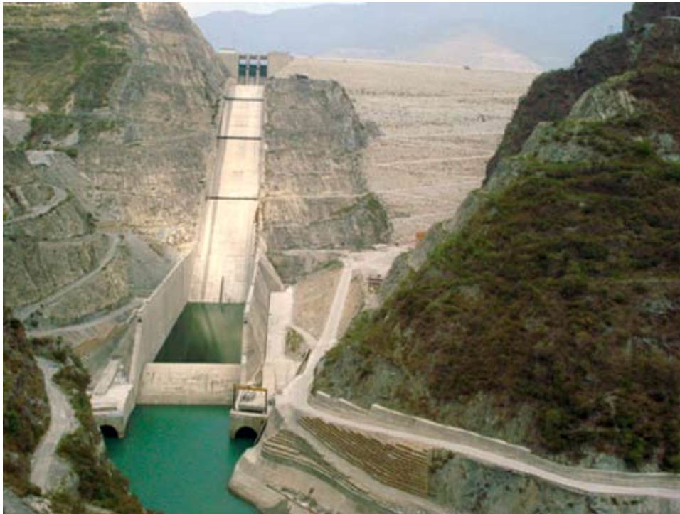
Tehri Dam/Arvind Iyer
