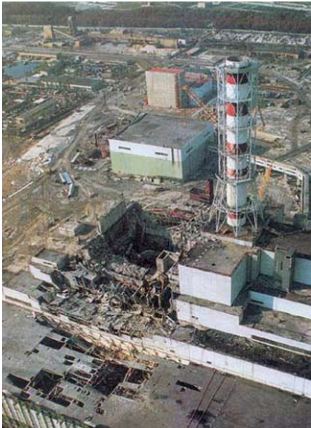
The aftermath of the 1986 Chernobyl accident, showing damage to the main reactor hall and the turbine building. This type of plant was never intended for electric power generation.
