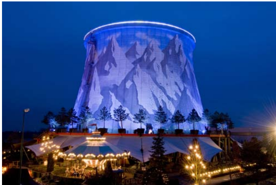
The fast-breeder reactor in Kalkar, Germany, was closed down in 1991 and turned into an amusement park. Its cooling tower is now a "climbing wall." Without reprocessing of nuclear fuel, Germany faces a cold, dark future.
