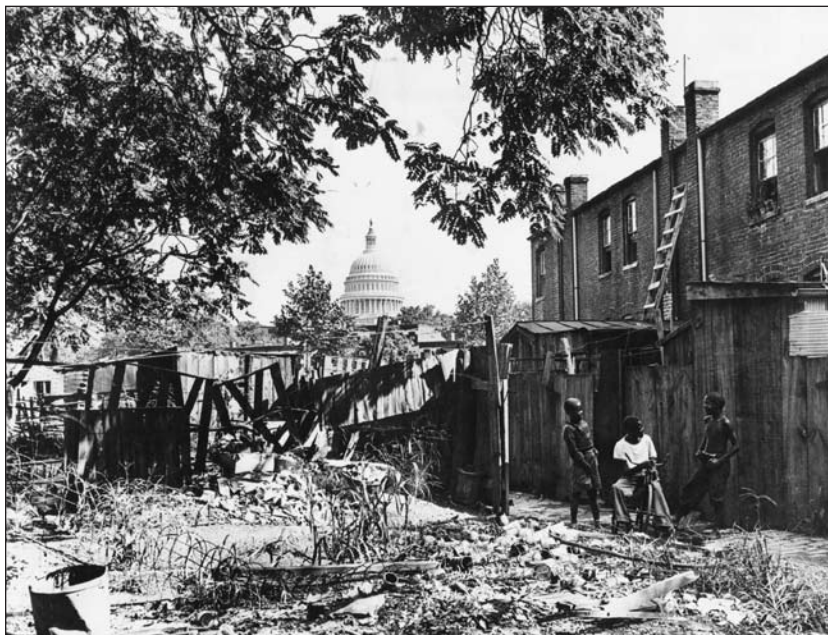
Conditions of squalor, like this pictured in Washington, D.C. in 1940, were the target of FDR's program of aid to localities under the Emergency Relief Administration. Today, we're headed back in the same direction, unless LaRouche's emergency actions are rapidly put into effect.
