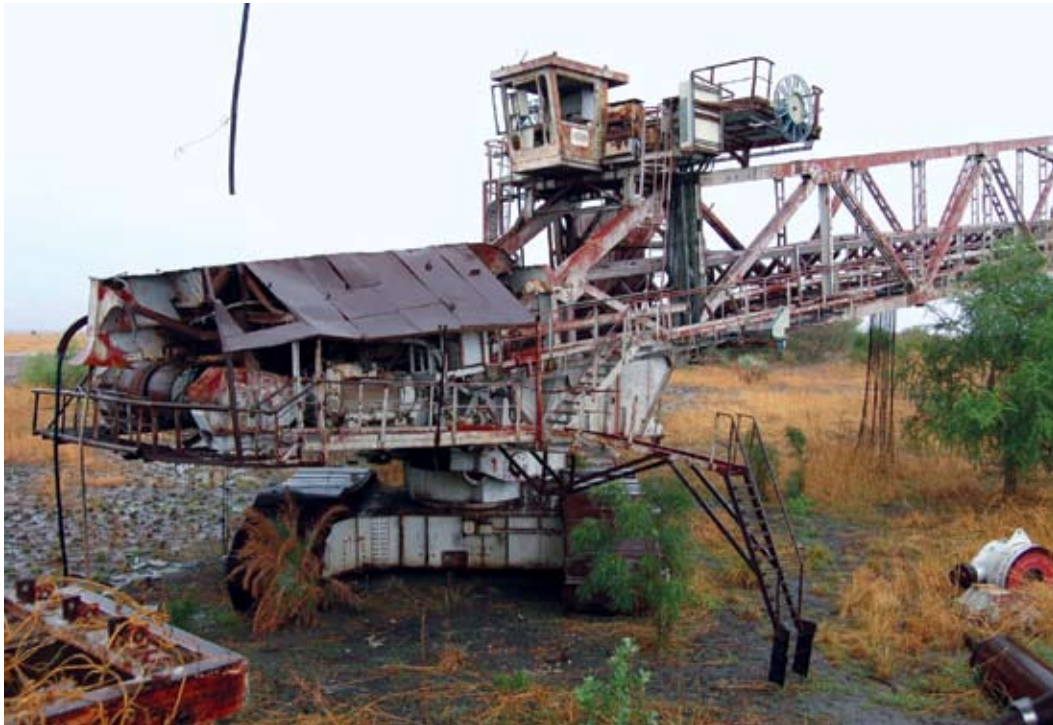
The Jonglei Canal project in Sudan was intended to create an agro-industrial renaissance for the region. In 1978, a huge German-built excavating machine, given the name “Sarah,” was brought in, which could dig 3 km in 10 days. But, in 1984, construction stopped, when Sudan People’s Liberation Army rebels started shooting at Sarah and the canal workers. This is Sarah today.
