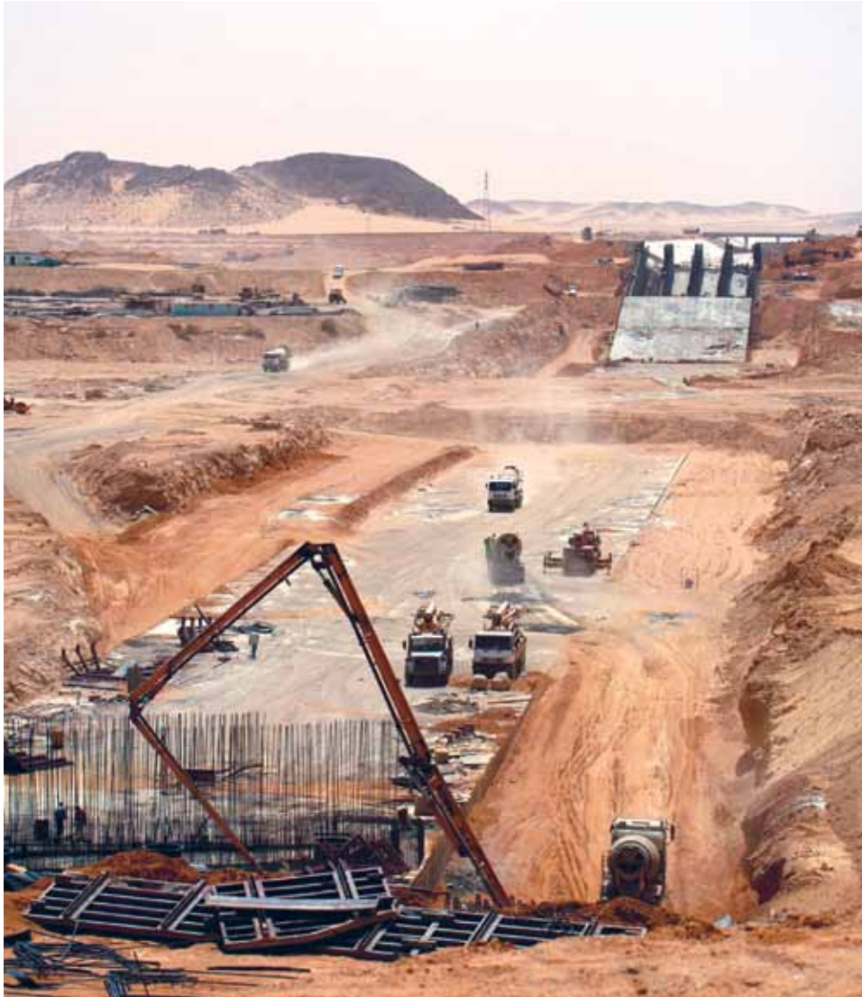
The Toshka Project, showing the construction site (2010) of the syphon that will deliver water to desert areas.
