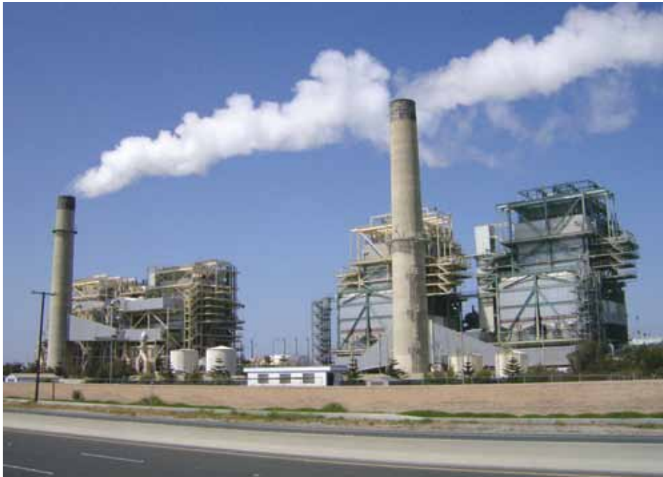
The unfinished Huntington Beach, Calif. desalination plant
