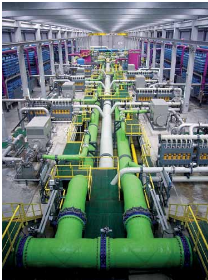
A Middle East reconstruction program for real development will require extensive desalination of sea water. Here, a reverse osmosis desalination plant in Barcelona, Spain.
