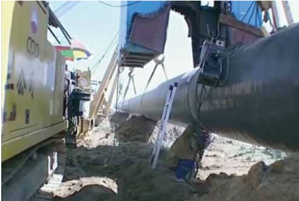
Laying the Central Asia-China Gas Pipeline's Line D across Tajikistan.
