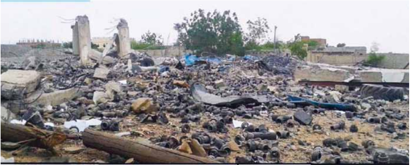
Destroyed water utility in Abbs, Hajjah, Yemen.
