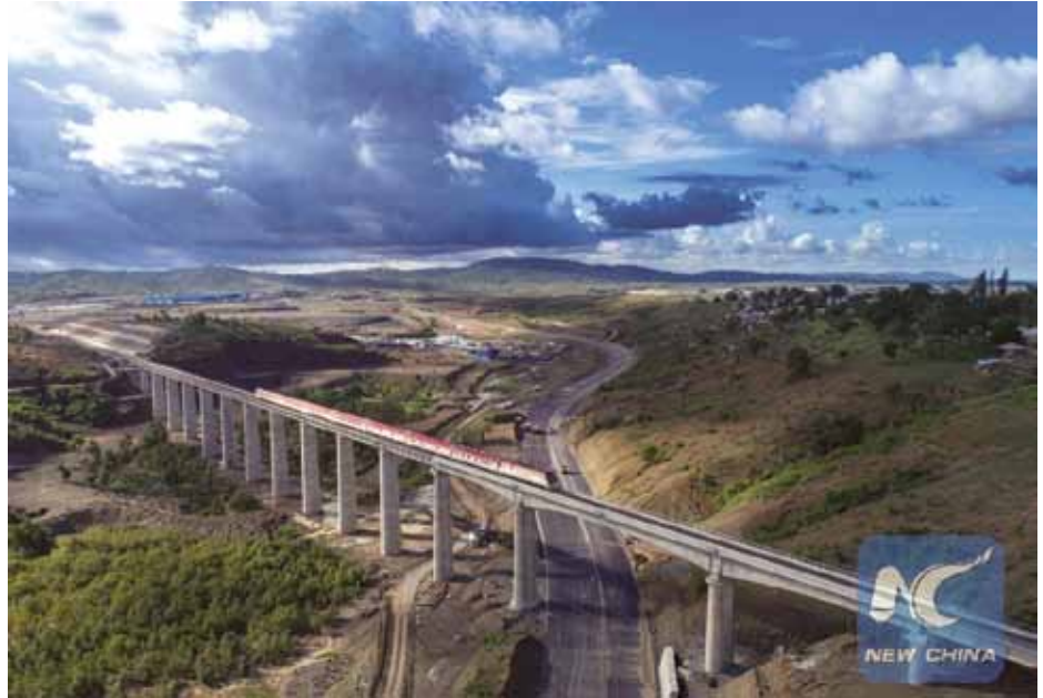
Chinese-built high speed rail in Kenya.
