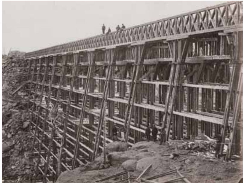
Andrew J. Russell/Yale University Collection Dale Creek Bridge during the construction of the Union Pacific Railroad, 1864-1869.
